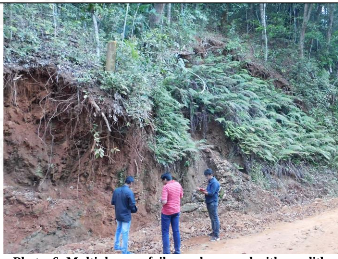
Photo 6: Multiple mass failures along road with regolith thickness >5m, NW of Terali, TS No. 48I/8
