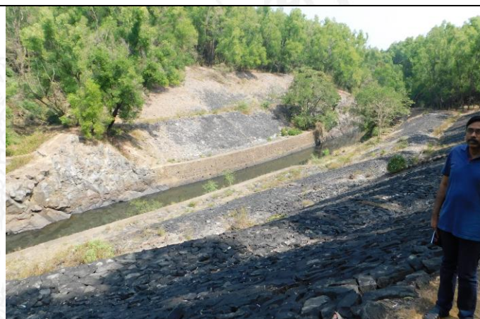
Photo 16: Transportational water Tunnel, Benching & Rock pitching provided for slope stabilization, East of Kumbharvada; TS No. 48I/8.
