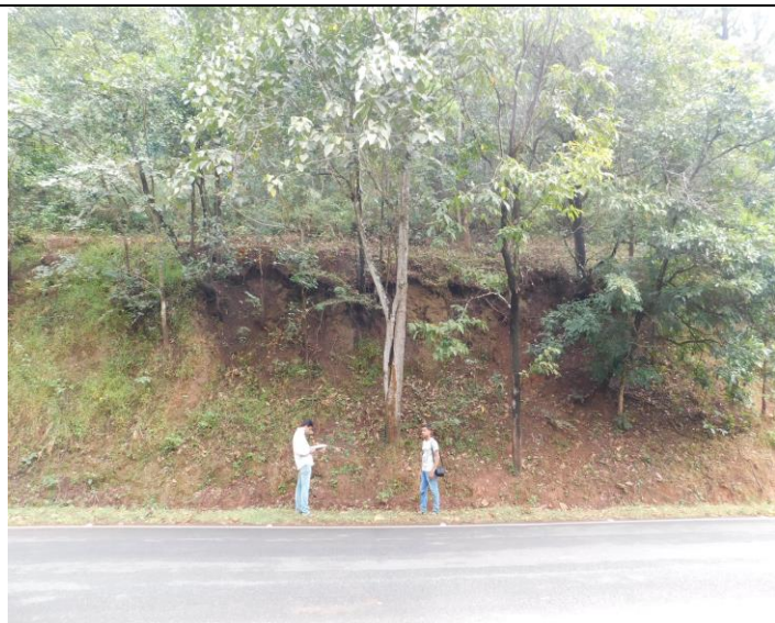
Photo 1: Extensive Cut Slope in in-situ soil. South-West of Usoda, TS No. 48I/11.
