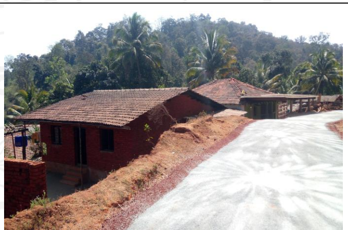
Photo 18: Settlements on modified slope observed in Vill. Chandrali, TS No. 48I/8
